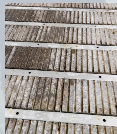
Figure 4: The photo shows strips in the slatted floor that separate faeces and urine at the source. The urine flows through the separation strips to the cellar while the faeces remain on top.
