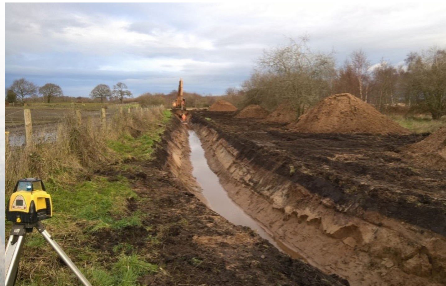
Figure 5: Photo showing the 2.9 km diversion route for the Bronington Manor Drain under construction to prevent nutrient-rich mineral water affecting core parts of the bog (Credit NE & WMP)
