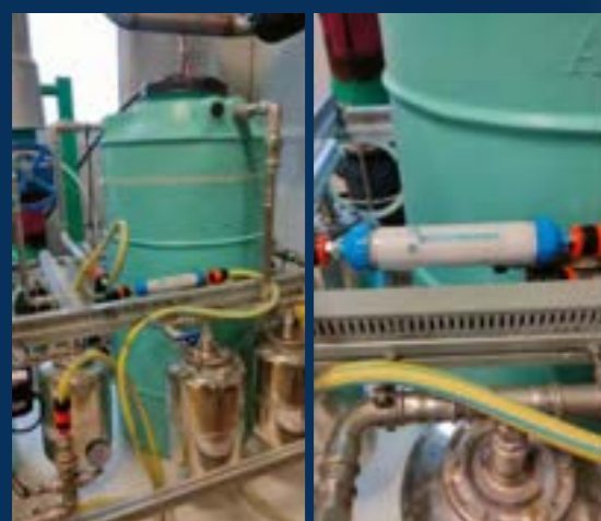
Figure 6: Pilot testing installation at Menù srl: food processing sector.
