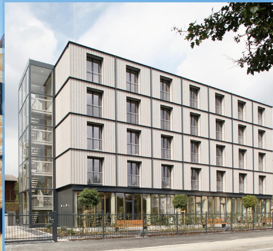
Schülerwohnheim Rehau, Germany: a five-storey school dormitory and canteen constructed completely from wood, including the lift shaft and staircase. Utilising a cost-effective modular construction, even inferior-grade wood was given value by using it for interior finishes.
