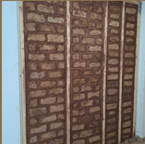
EcoTechWall – South European type with light clay bricks.
